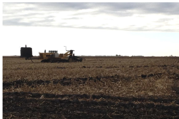
Figure 1. Subsurface drainage installation
